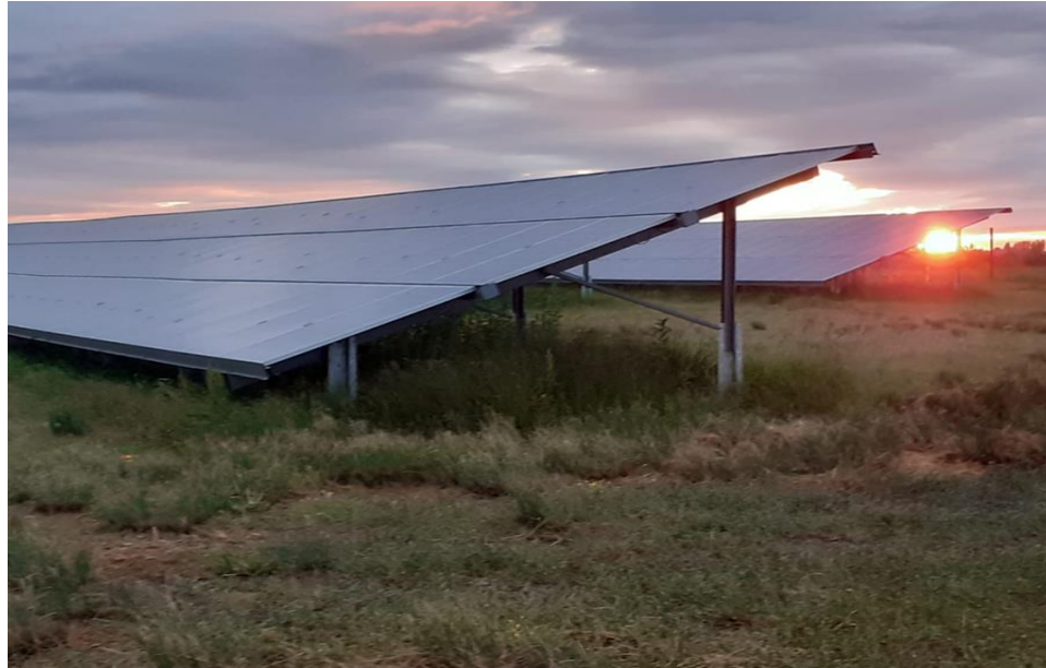
Photo of solar panel at Gedling County Park
